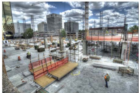
Construction of the new County Courts Building
